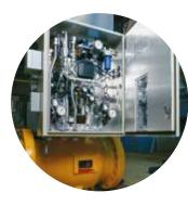
Integrated control arrangements Each control valve will be supplied with integrated fit-for-purpose control arrangement.
