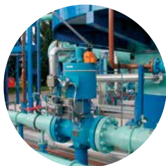
8" / ASME 600 Axial Control Valve
