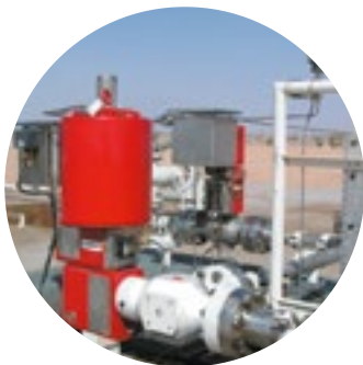
4 1/16" / API 5000 Angle Choke Valve
