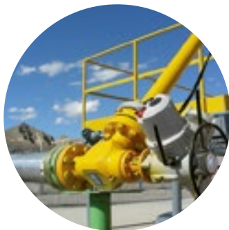
3" / API 15 000 Angle Choke Valve
